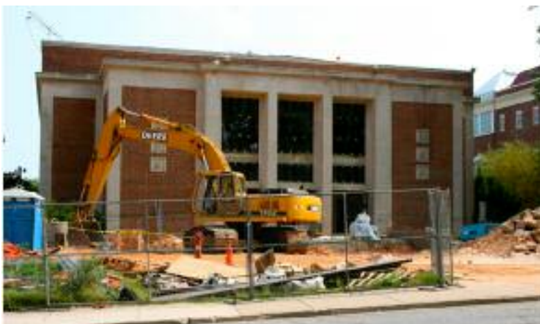
Jarman renovation as of July, 2010
