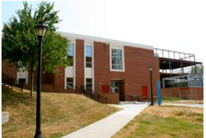
New Wygal elevator with the Bedford addition construction in the background
